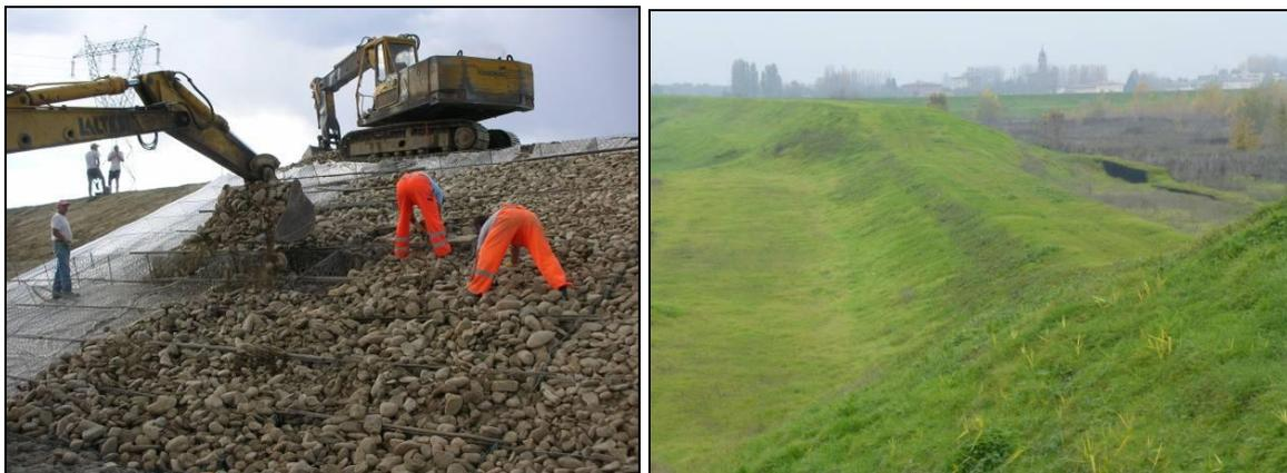
Figures 5, 6: the gabion spillway during construction and today
