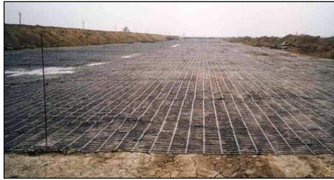
Figure 4: Installation of the reinforcing geogrids
